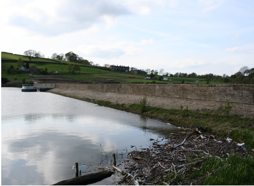
Figure 5: Hewenden Reservoir – Completed Wave Wall
