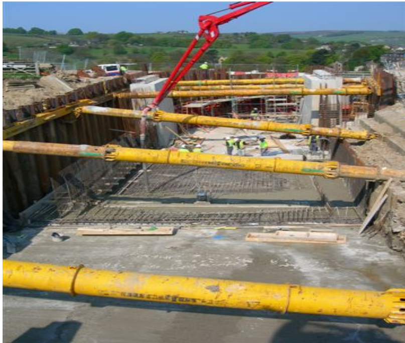
Figure 2: Tumble bay under construction
