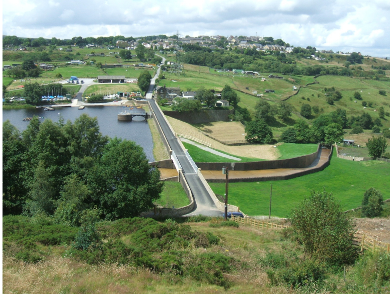
Figure 4: Doe Park Reservoir - Overview post construction
